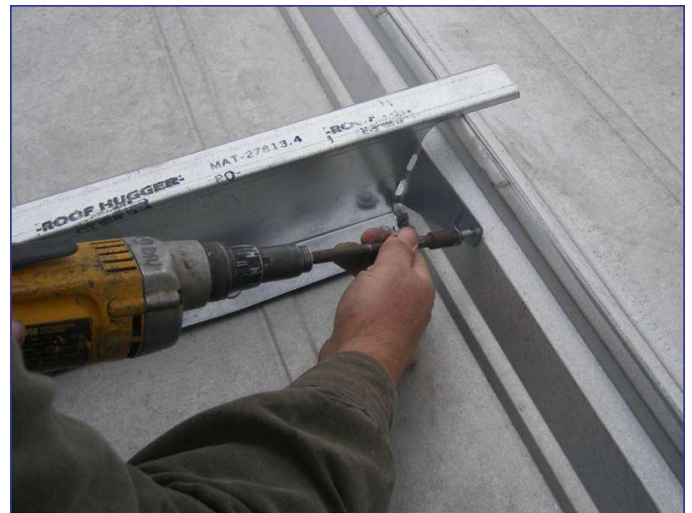
Anti-Rotation Arm Being Attached
