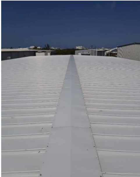
Finished Roof Ridge
