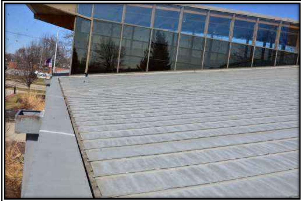
Photo D: This shop fabricated standing seam roof panel is composed of terne coated stainless roof panels with machine locked seams.
