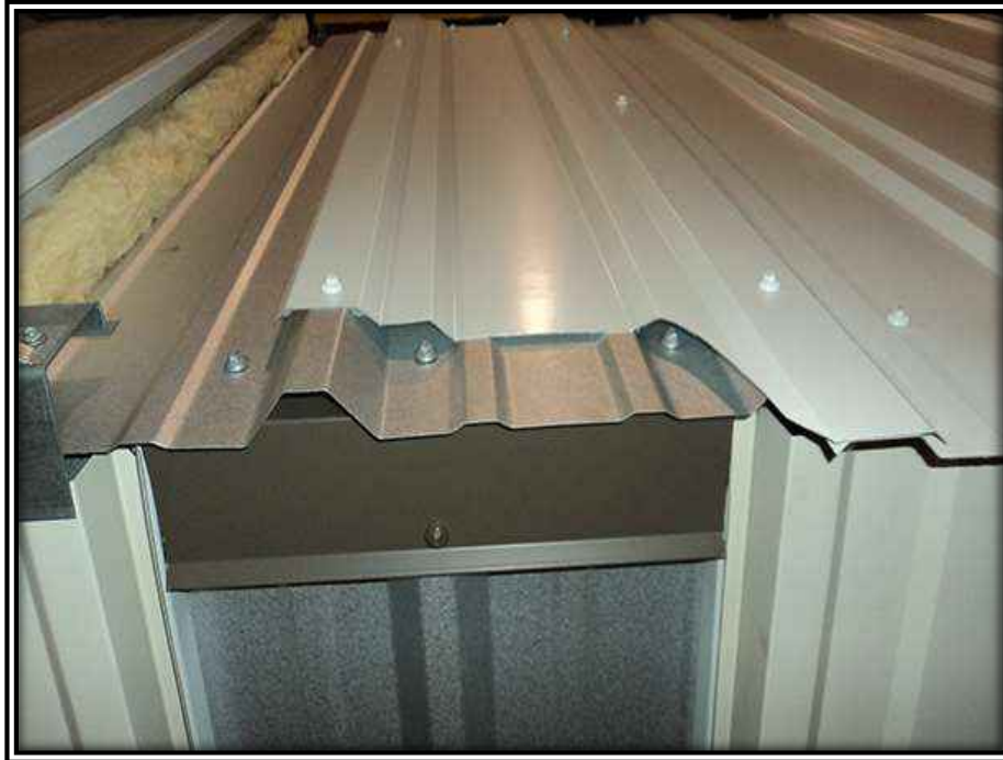
Photo J: A direct panel overlay as seen in the photo above is easily accomplish with “R” Panels.
