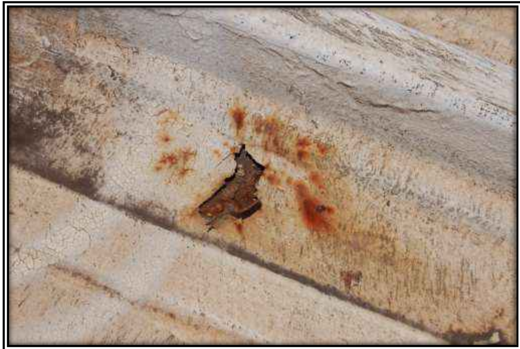
Photo F: Coatings that de-bond from the metal below can crack, allowing water to enter in below the coating and deteriorate the metal panel below.
