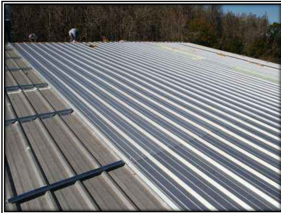
Photo K: Notched purlins placed over the existing standing seams in line with the purlins below is an efficient method to install a new roof panel.
