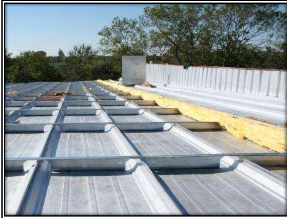
Photo L: Here a tall clip is being use in association with the notched purlin so that insulation can be incorporated into the new roof system.
