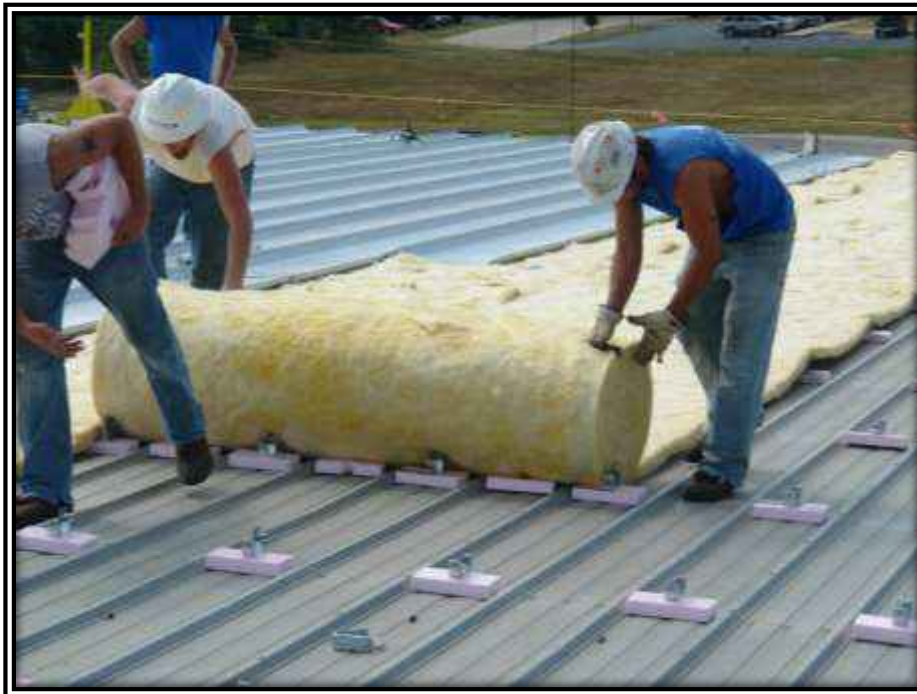
Photo M: Tall clips are being used to raise the height of the roof panel so that a layer of insulation can be installed.
