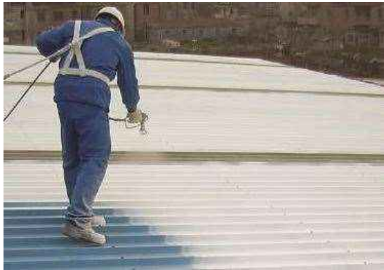
Spray applied Coating Metal over Metal Retrofit
