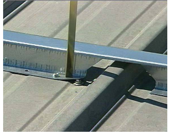
Existing fasteners usually do not have to be removed
