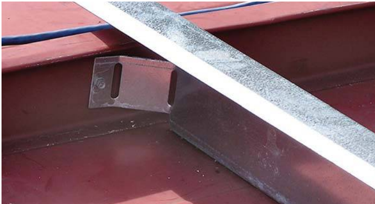
New Trapezoidal standing seam being installed over an old Vertical Rib standing seam with stand-off clips.
