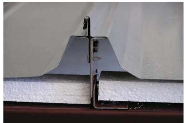
Typical standoff clip assembly for trapezoidal standing seam panel.
