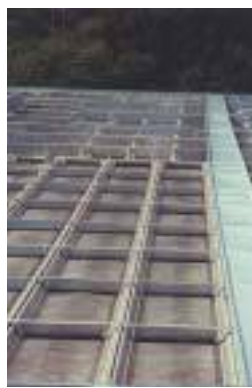
Roof Huggers in place on an old roof.
