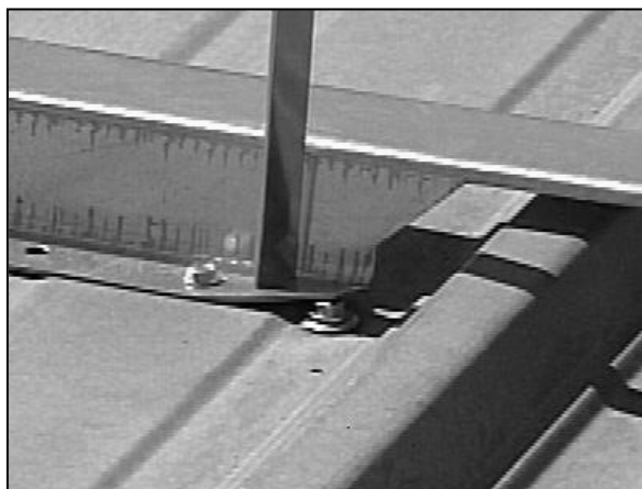
(Typical “R” Panel installation showing the bending of the bottom flange caused by the existing fastener is normal.)
