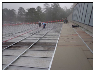
Rigid Board Insulation
