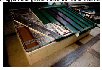
concealed clip attachment also means there is a minimal number of exposed fasteners penetrating the roof. High "R" value fiberglass or rigid insulation roof assemblies are possible and with standing seams roofs the insulation does not need to be fully compressed over the purlins, as is the case with screw down panels.
