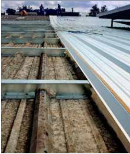
Retrofit framing over an existing roof
