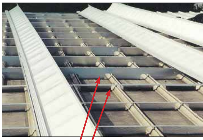
Using 2 different heights of ROOF HUGGERS to remove a roof "step".
