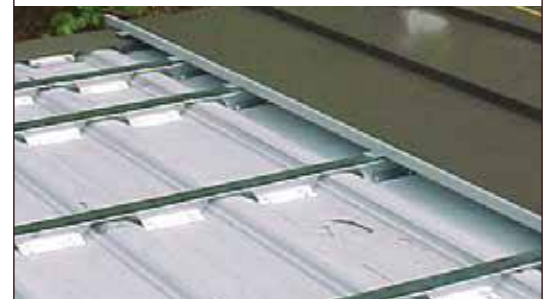
Vertical Rib Standing Seam over "R" Panel
