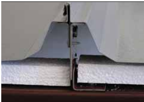
Typical high-clip assembly for trapezoidal standing seam panel.
