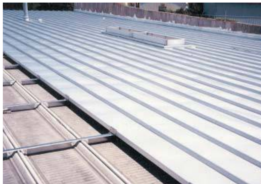
New panels being installed over Roof Huggers on an old roof (above).
