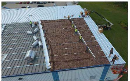
are not working over open framing which requires more equipment while exposing them to increased fall hazard, they are working on top of the existing roof. This makes stacking of material, equipment, tools, etc. much faster and easier.
