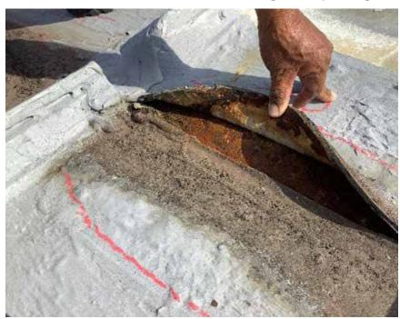
is questionable. The quoted material life ranges from 10-to-18 years with proper maintenance but, like regular coatings, if water becomes trapped between the coating and panel, the panels will corrode quickly and may become unrepairable.
