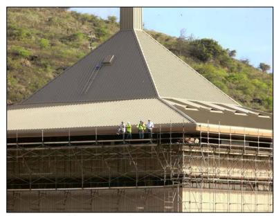
the other hand, architectural applications are commonly roofs with a slope of 3:12 or greater where the roof is being replaced for not only performance reasons but for aesthetic purposes as well.
