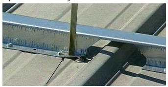
Typical "R" Panel installation showing the bending of the bottom flange caused by the existing fastener <u>is normal</u>.
