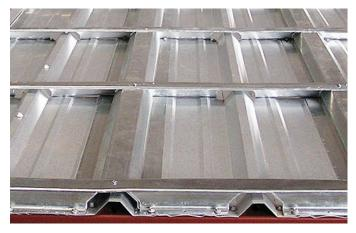
Note: If integral (fit under the HUGGERS) structural Sub-Rafters are provided, loosely place hats and HUGGERS in position prior to installing any fasteners to prevent alignment problems in these areas.
