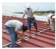
ordered with a narrower starter panel to offset the new panel from the existing panel module. If landing on the cut ends is unavoidable then attach the adjacent HUGGERS overlapping top flange ends with (2) #10 pancake head fasteners in addition to the clip fasteners or back lap the HUGGERS one full corrugation to produce a double thickness and continuity of the top flange across the lap.
