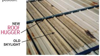
Cut out and trim opening if new skylights are to installed above, or leave panel in position if skylights are to be eliminated. Removal of skylight prior to installing HUGGERS may result in an undesirable depression of the new roof over the old skylight area.
