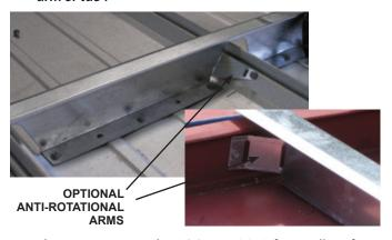
This arm prevents the ROOF HUGGER from rolling front to back under load and it is attached with a #17 fastener into the side of the existing panel high rib. Note that if the anti-roll tab is above the side of the existing high rib the ROOF HUGGER may not be pulled fully down into its correct position.
