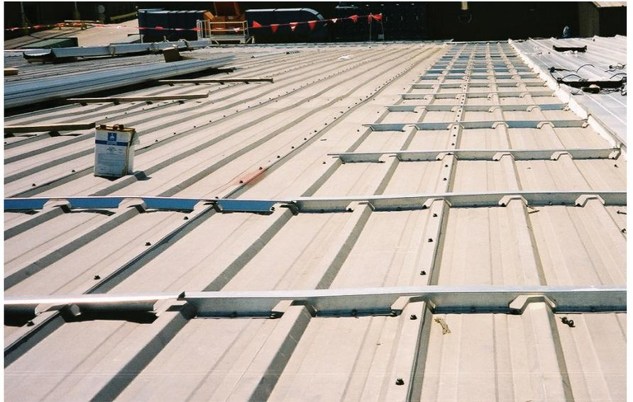
*JG Smith Construction tried different methods of installation, but found the Roof Hugger to be the most efficient metal roofing retrofit system for its uses at the Mills Pride furniture manufacturing complex in Waverly, Ohio. JG SMITH CONSTRUCTION PHOTOS*
