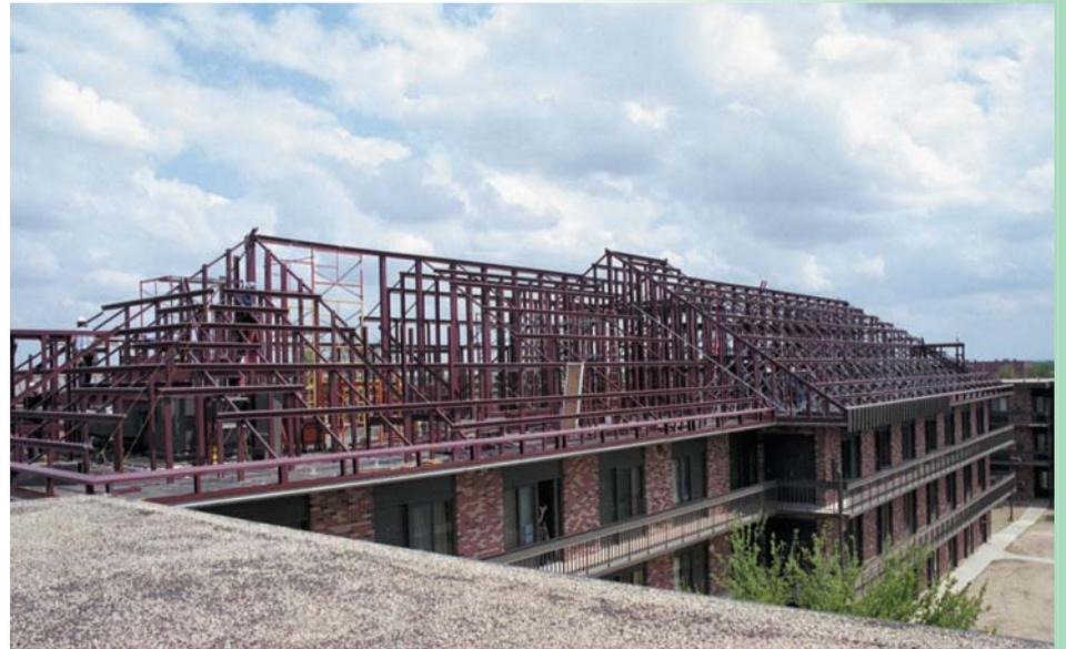
Reroofing offers tremendous market potential, whether building slope over a flat roof (as shown above) or retrofitting an old thru-fastener metal roof with the Roof Hugger system (demonstrated below).
