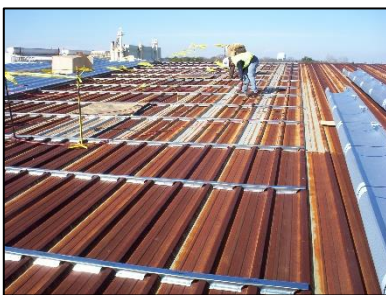
Model "C" ROOF HUGGER Sub-Purlin System installed over existing exposed fastener Ribbed Panel with new Trapezoidal Rib SSR. Also, available for existing 6" to 10" rib spacing.
