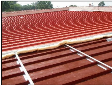
ROOF HUGGER Sub-purlin for existing Vertical Rib standing seam panels with new Trapezoidal Rib SSR.
