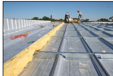
ROOF HUGGER Sub-purlin for existing Trapezoidal Rib standing seam panels with new Trapezoidal Rib SSR.
