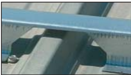
A closer view of a Roof Hugger after installation.
